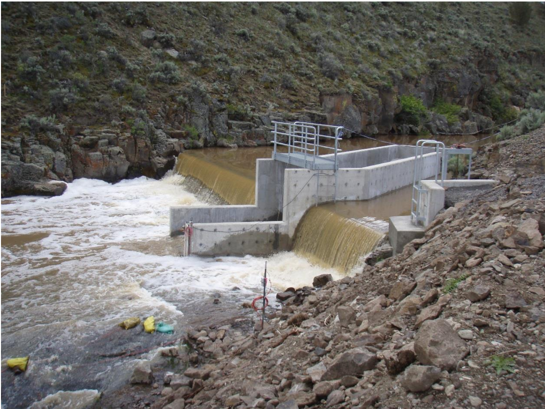
Photograph of the Dike Diversion and fishway on lower Twentymile Creek during a May 2015 freshet.
