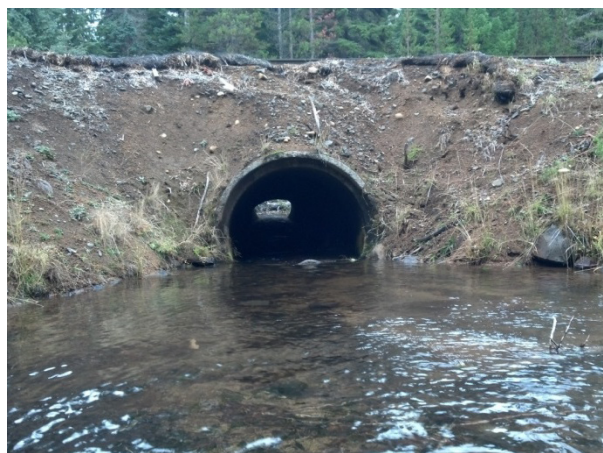
FIGURE 1.17—Railroad culvert (27 m long) on Crystal Creek; upper panel looking upstream, lower panel looking downstream.
