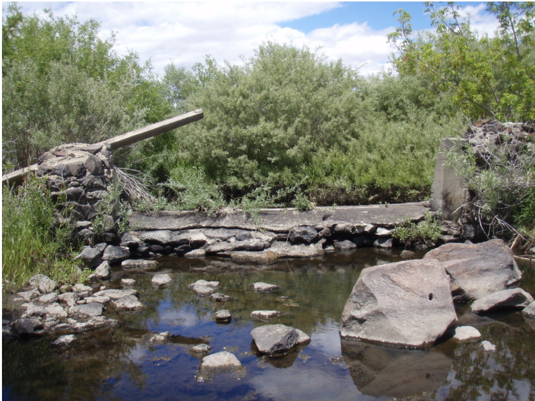
Photograph of an aging irrigation diversion structure on lower Honey Creek.
